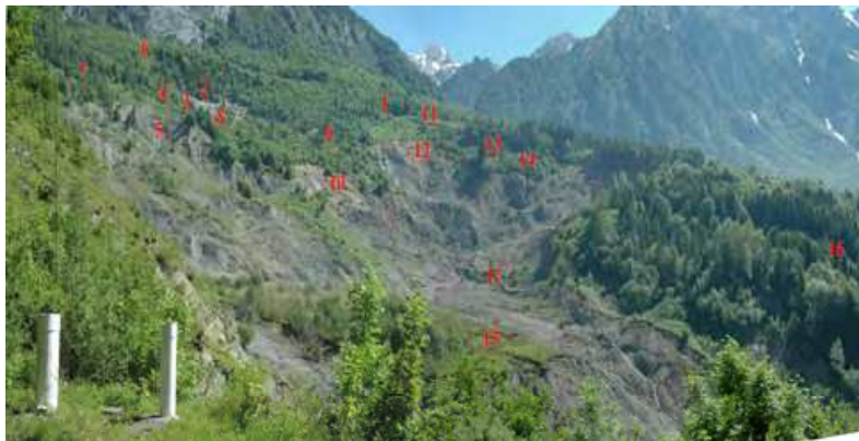
Fig. 5. View from the radar installation of the monitored area. Red figures indicate benchmarks for optical measuring (After Luzi et al., 2006).
