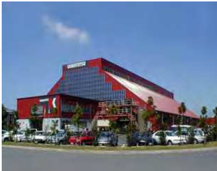
Photo 2. MSW gasification plant in Chiba (Japan)
