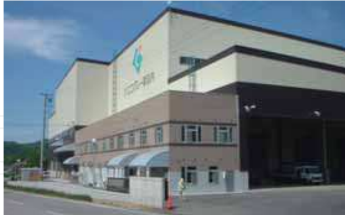
Photo 3. “Plasma Assisted” gasification unit owned by Hitachi Metals with treatment capacity of 200 tones of municipal solid waste and automobile shredder residue per day in Utashinai in Japan (Circeo, 2007)
