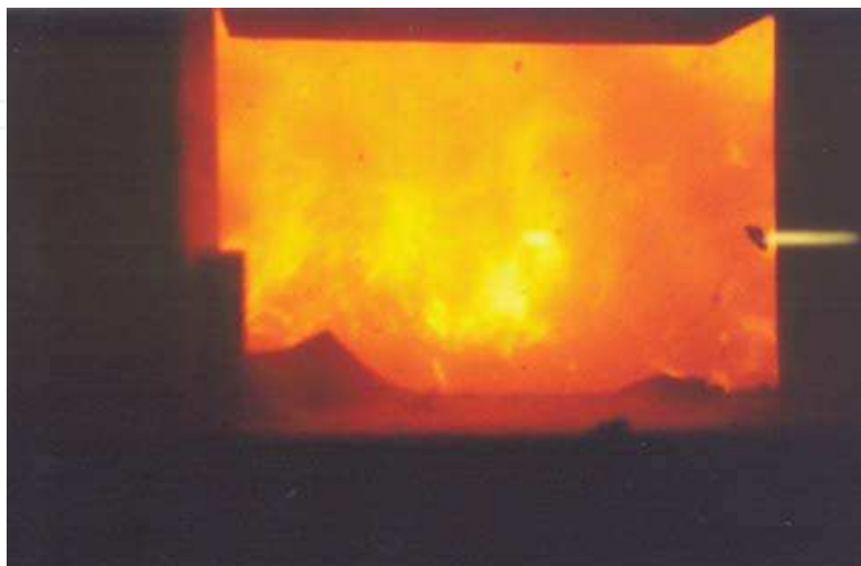
Fig. 3. Inside of an incineration chamber in Valorsul's incinerator (S. João da Talha, Loures, Portugal).
