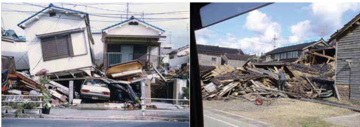
Fig. 1. Collapsed Japanese wooden houses in Kobe (1995, the left figure) and Noto (2007, the right figure) earthquakes
