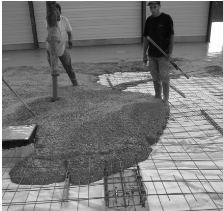
Fig. 10. Sensor cable must be robust: example of concrete pouring . Extracted from (Dubois et al., 2007)
