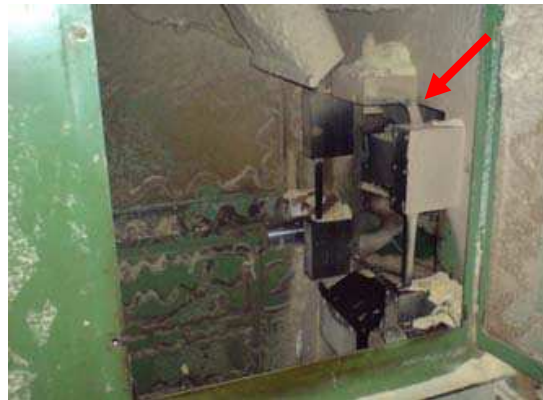
Fig. 10. Antenna for RFID reading in the sawline. The arrow is indicating the position of the antenna.
