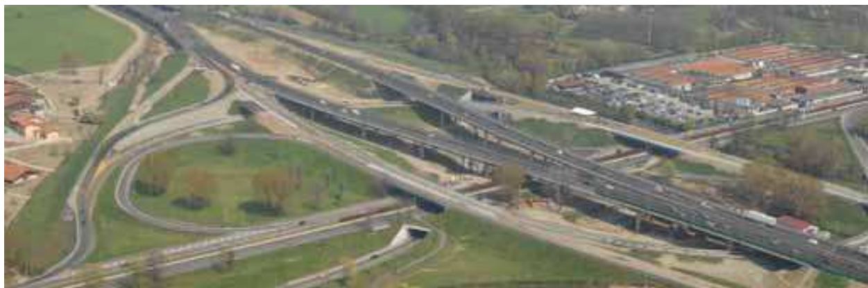
Fig. 12. Aerial view of the new viaduct over Forlanini Avenue, Milan, Italy
