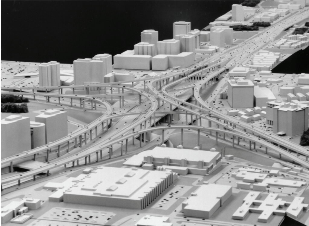
Figure 6. Dallas High Five interchange (source http://www.dallashighfive.org . November 2003)
