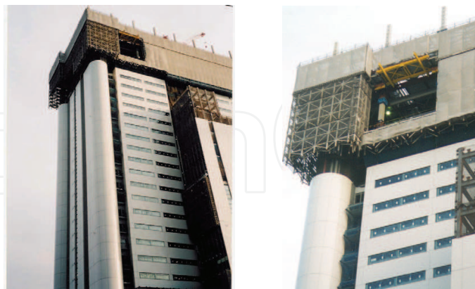
Fig. 1. An automated construction system in Japan.
