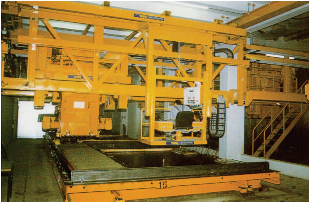
Fig. 4. Teleoperated concrete distribution
