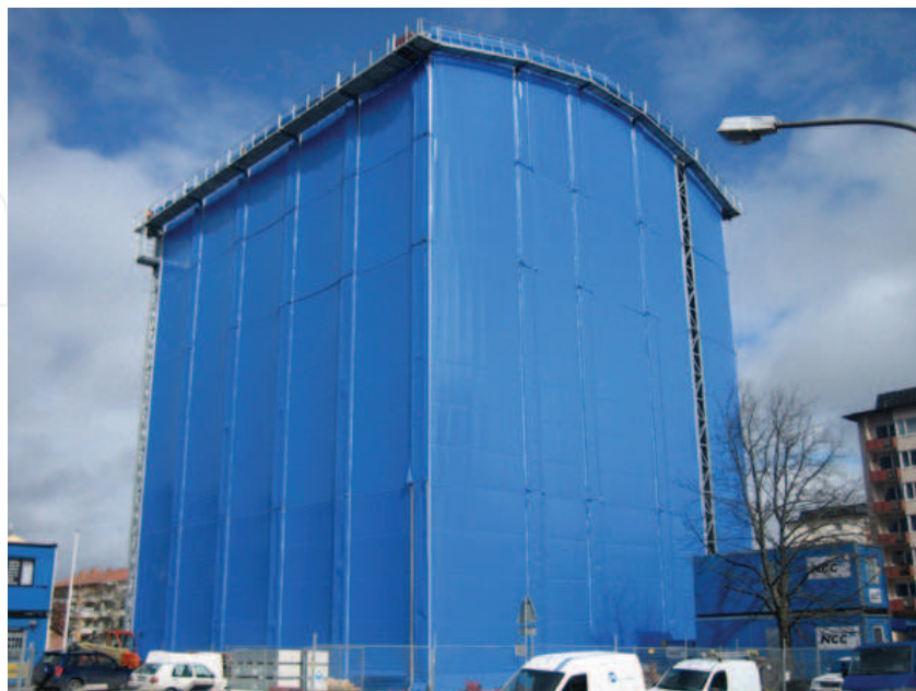
Fig. 11. On site factory of NCC Komplet
