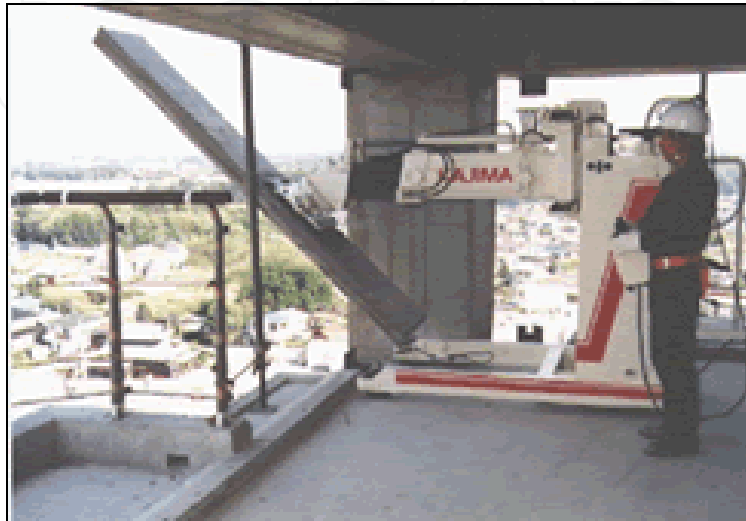
Fig. 7. Kajima's interior wall assembly robot
