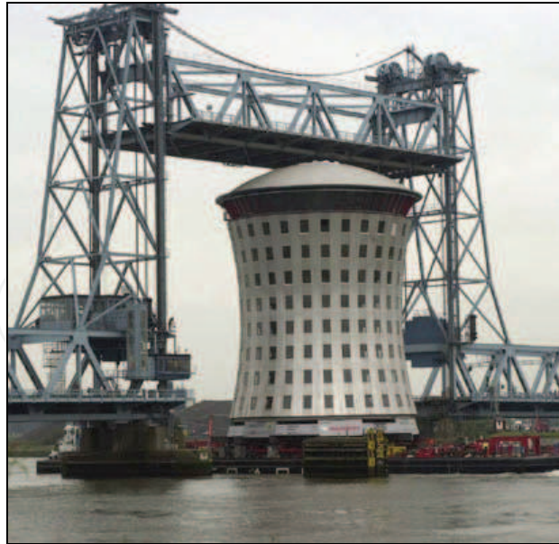
Fig. 13. Bolder building transportation by water
