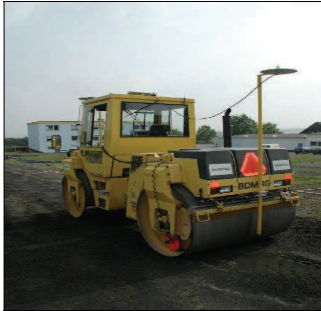
Fig. 3. OSYRIS project sensor-based compactor
