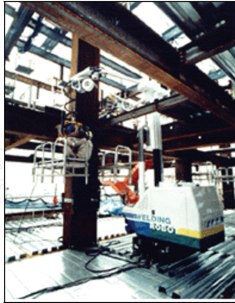
Fig. 11. WR mobile robot for column welding
