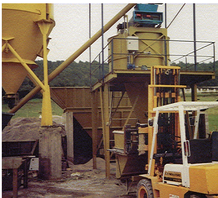
Fig. 5. The materials feeding and mixing platform
