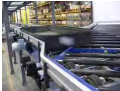
Figure 7. A diverter element with an empty oversize tote
