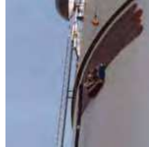
f) Hydro-Crawler working
