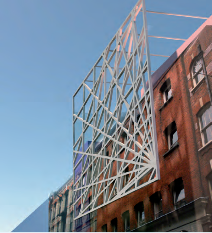
showing the structure cantilevered over the fascia provide a sun baffle.
