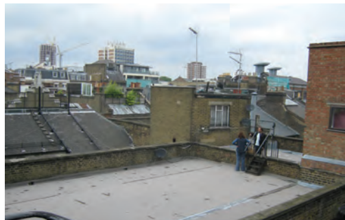
ROOFTOP facing at Charlotte Road
