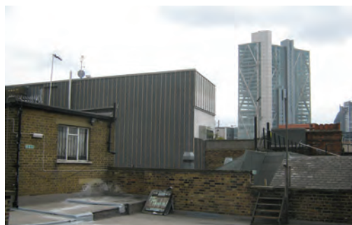
ROOFTOP facing the middle platform
