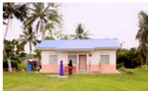
Figure 4: Surroundings of the low-cost location single story detached house used for field measurement.
