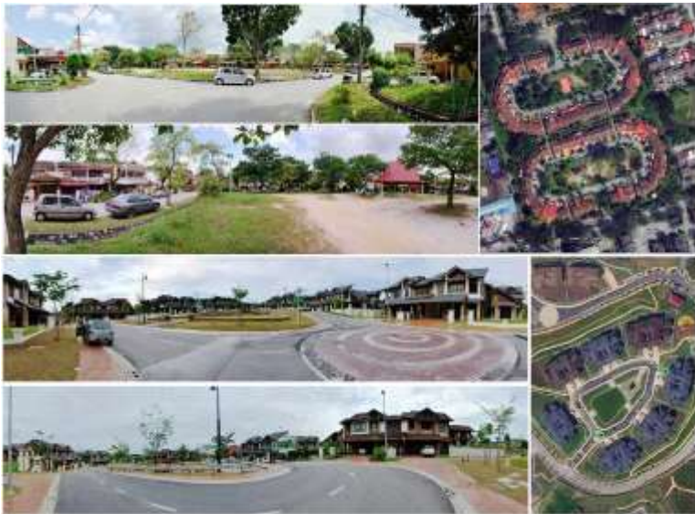
Figure 1: Technical Visual Analysis of Seksyen 18/5A, 14A and U8/74C. Exemplifying the stark contrast of varying cul-de-sac courtyard arrangements and typology. Top right: Google Earth from 509m Eye Altitude of Seksyen 18. Top cul-de-sac – 18/14A, bottom cul-de-sac – 18/5A with corresponding panoramas. Bottom Right: Google Earth from 521m Eye Altitude of Seksyen U8/74C (Bukit Jelutong), with panoramic street approaches into the cul-de-sac courtyard (left) (4th October 2011).
