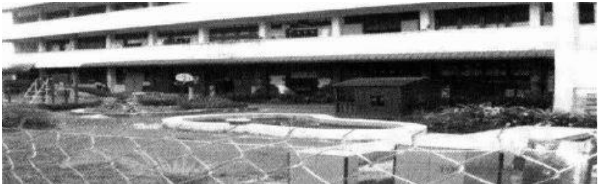
Figure 2.2: Front view of renovated existing public preschool classroom
