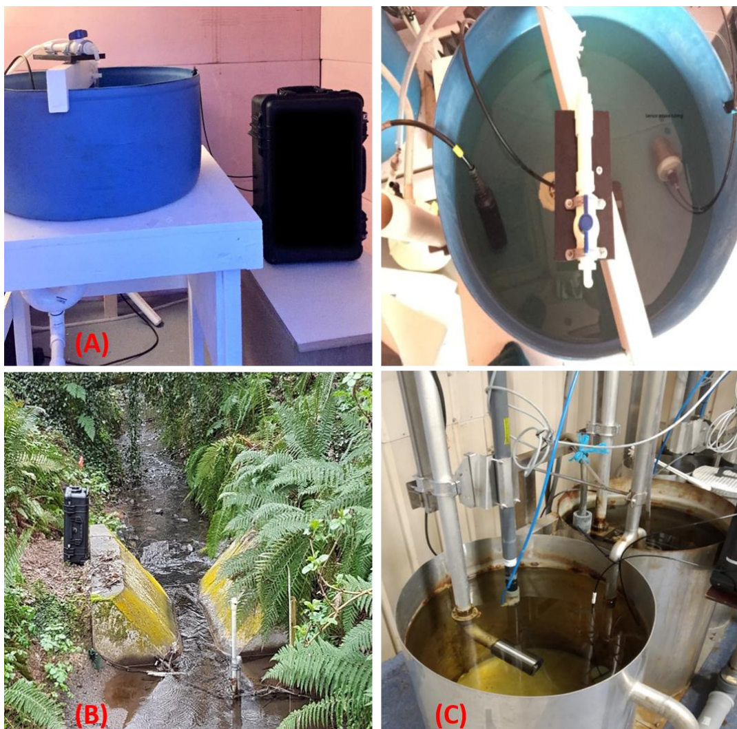
Figure E1: (A) Photograph of the portable IC system deployed in the US and picture of the water test tank. (B) Photo of system deployed in Teagasc Johnstown Castle analysing surface water. (C) Photo of portable IC system sampling from process water at effluent treatment plant in Haapavesi, Finland.
