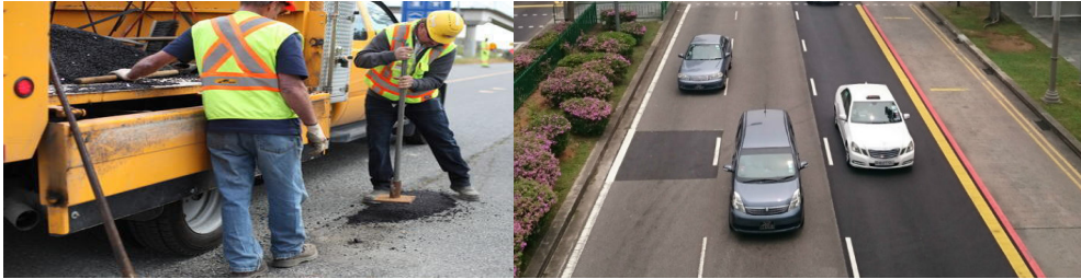
Figure 6: Prompt road maintenance on site
