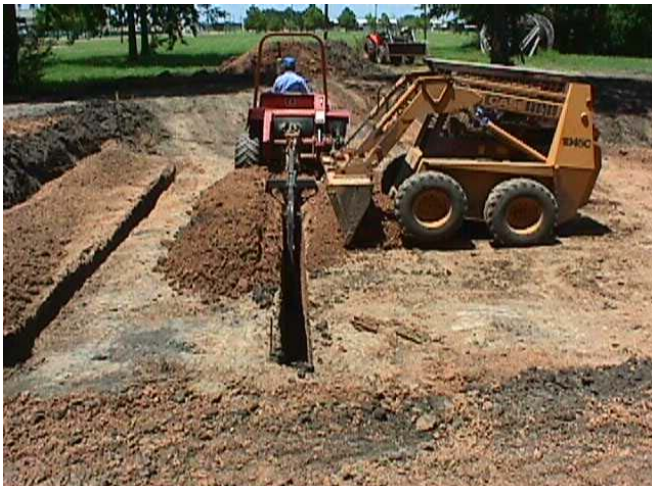
Figure 3.6. Test Module Fin Construction.
