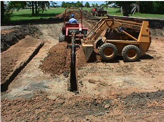
Figure 3.6. Test Module Fin Construction.
