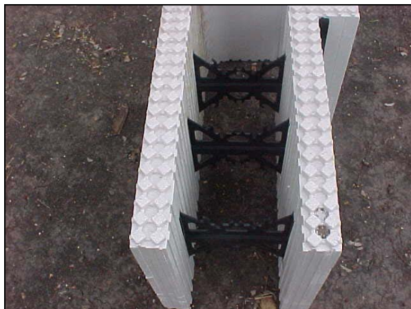
Figure 4.3. ICF Units with Spanners
