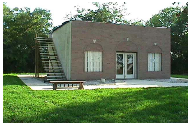
Figure 3.11. Finished Test Module.
