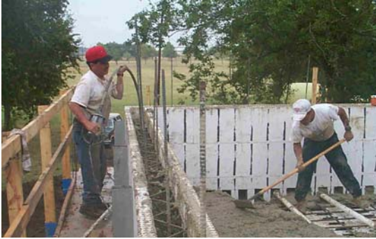
Figure 3.9. Placement of Test Module Concrete.
