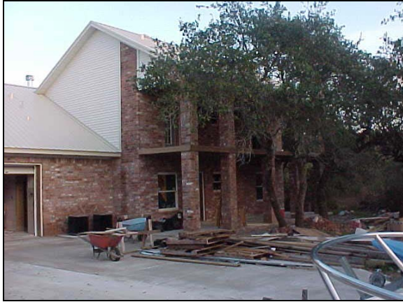
Figure 4.5. Rear View, Showing Second Floor
