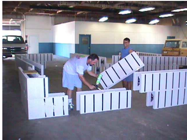
Figure 3.5. Forms Provided by ARXX Building Systems.
