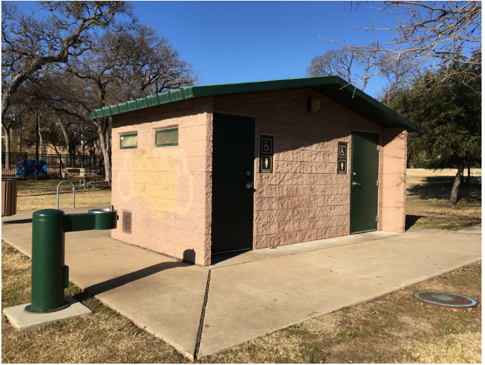
Figure 4.68 shows bathroom conditions
