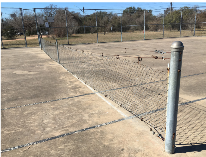
Figure 4.20 Shows a chain link fence used as a net
