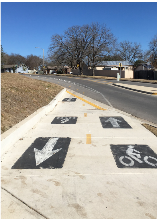
Figure 4.44 shows bicycle lanes at Ponciana Park
