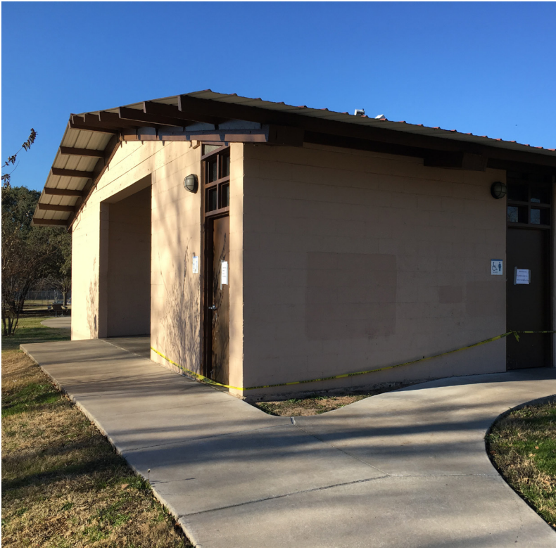
Figure 4.59 shows closed bathroom
