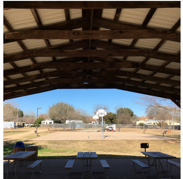
Figure 4.40 shows Franklin Park pavilion
