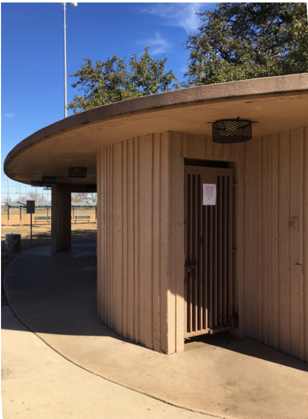
Figure 4.23 Shows the locked door at only bathroom
