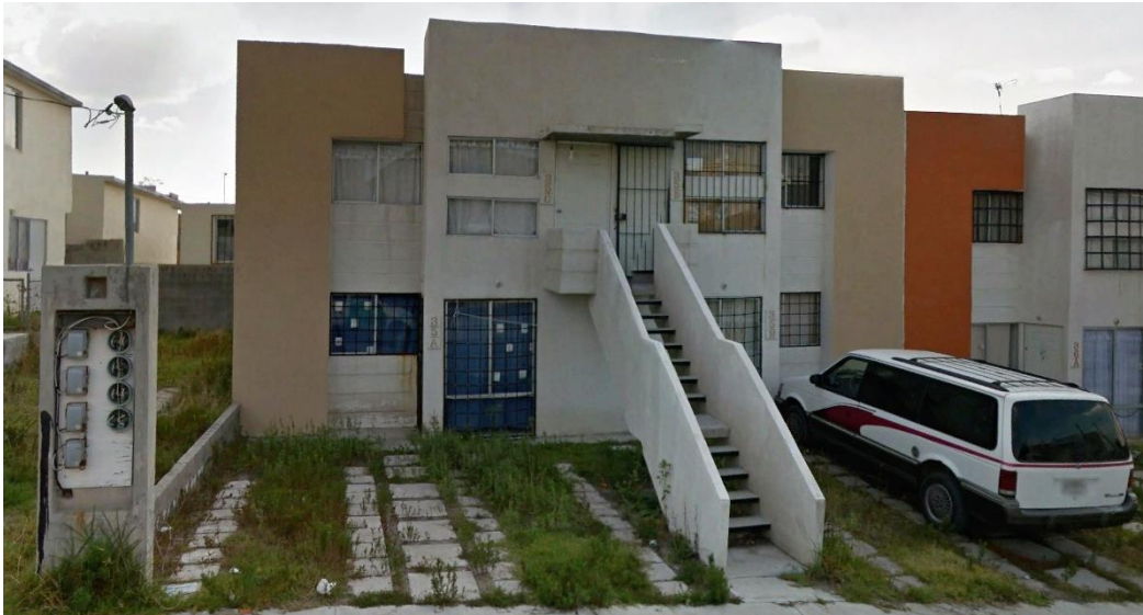
Figure 5.33: Multi-family Housing with No Electricity Meters in Santa Teresa, Huehuetoca.
