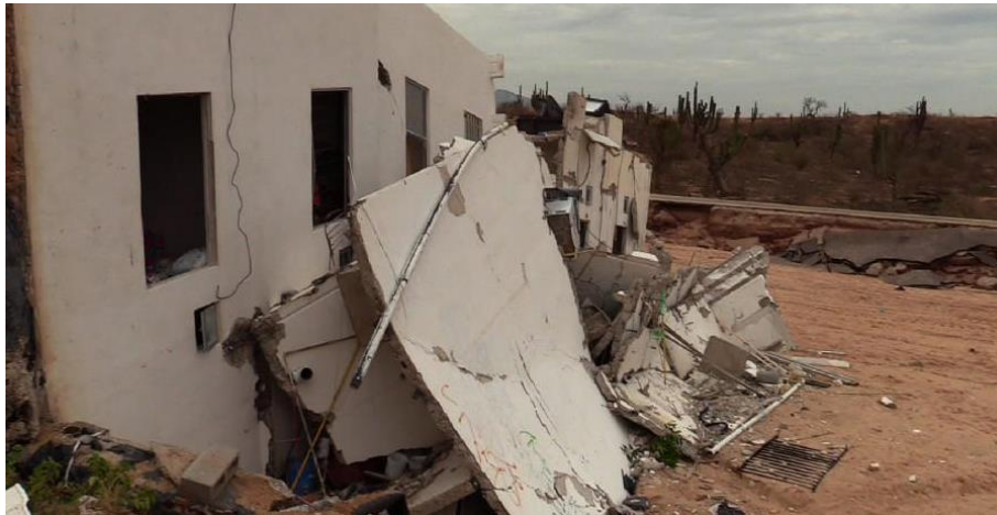
Figure 5.8: Colapsed Homex Development in Cabo San Lucas, Baja California Sur.
