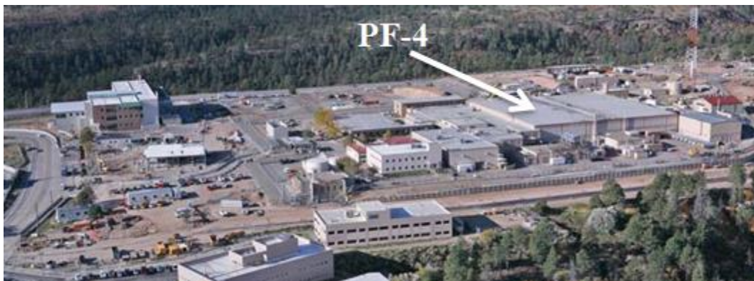
Figure 6-6. Plutonium Facility (PF-4) at LANL. [LANL, 2013]
