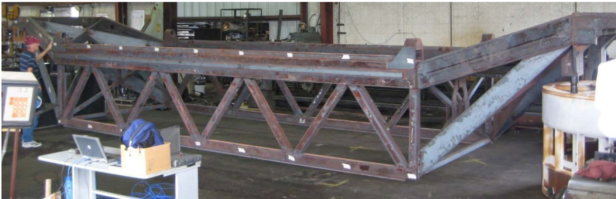
Figure 11: Photograph of the bridge after completion of fabrication and stress relieving, prior to machining
