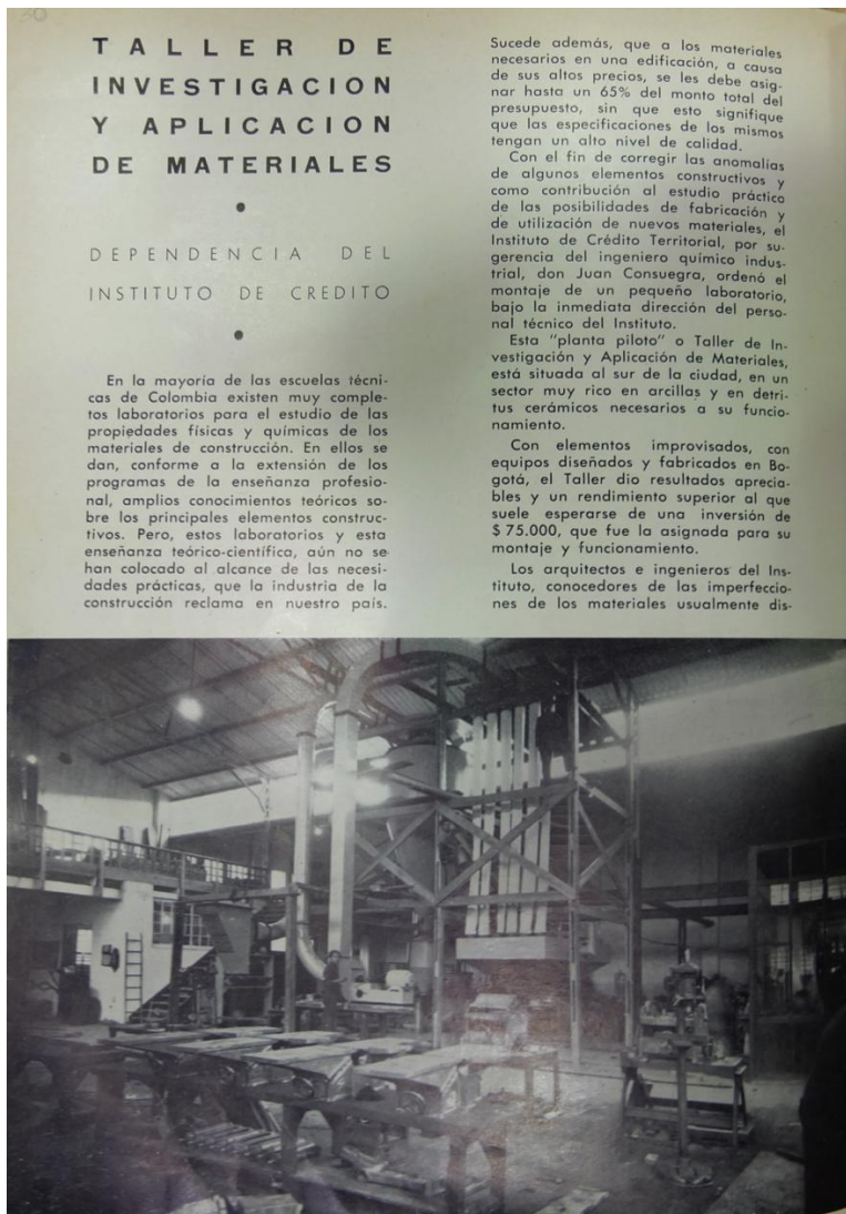
Figure 3.5. Materials Application Workshop, Proa 28. October 1949.
