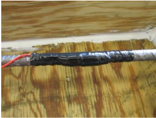
(e) Duct tape finishing
