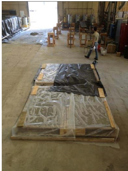
(h) After concrete casting
