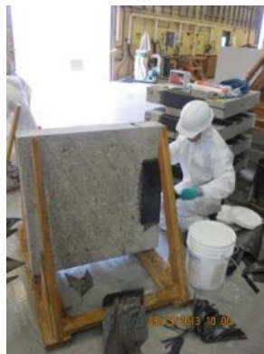
(e) Attaching CFRP strip to concrete surface
