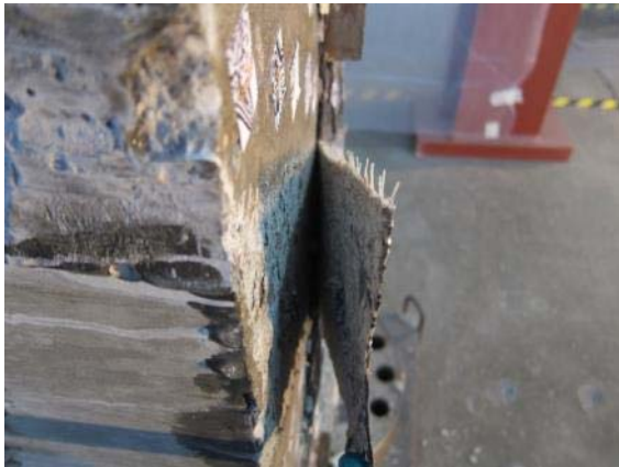
(c) Failure mode of B5-60-0-5
