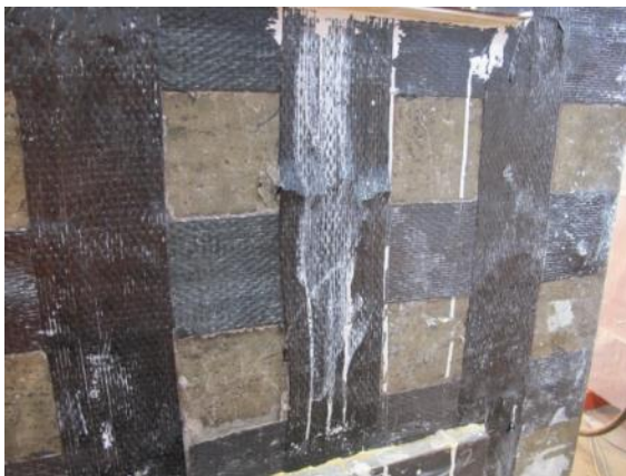
(c) Failure mode of B5-0-0-5
