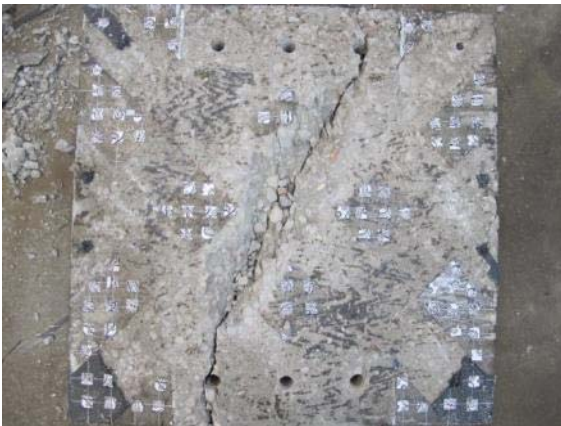
(e) Crack pattern of B5-45-0-5
