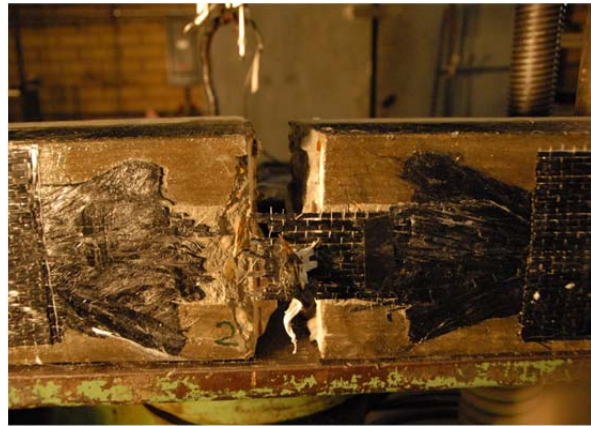
(b) CFRP strip rupture
