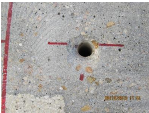
(c) Rounding the edge of the hole
