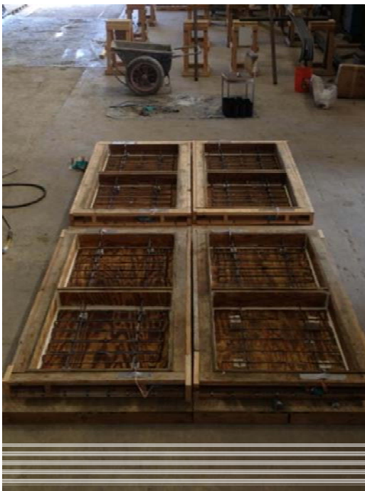
(g) Rebar mats in the wood forms
