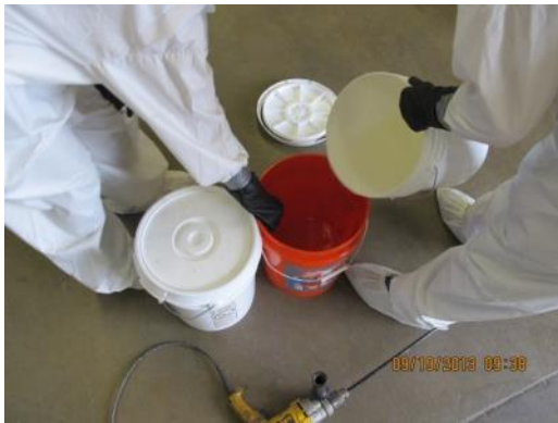
(a) Mix component A and B
