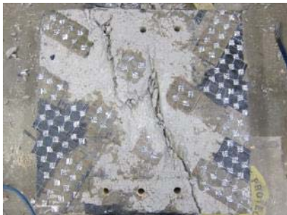
(c) Crack pattern
