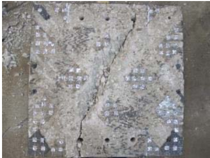
(c) Crack pattern
