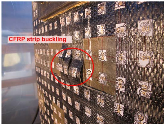
(c) Failure mode of B5-0-0-5
