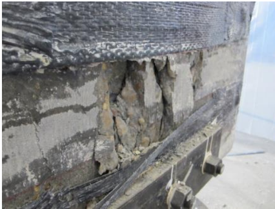
(c) CFRP strip failure of U5-0-1-5
