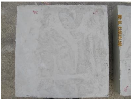
(a) Removal of forms
