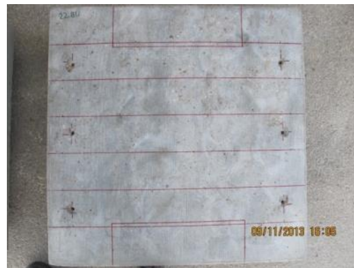
(b) Concrete surface grinding
