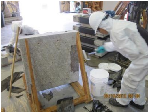
(c) Saturating the concrete surface
