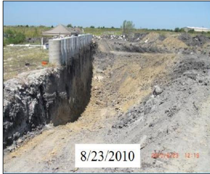
Figure 6.13: 1:1 Slope excavation to the depth of 15ft (8/23/2010)
