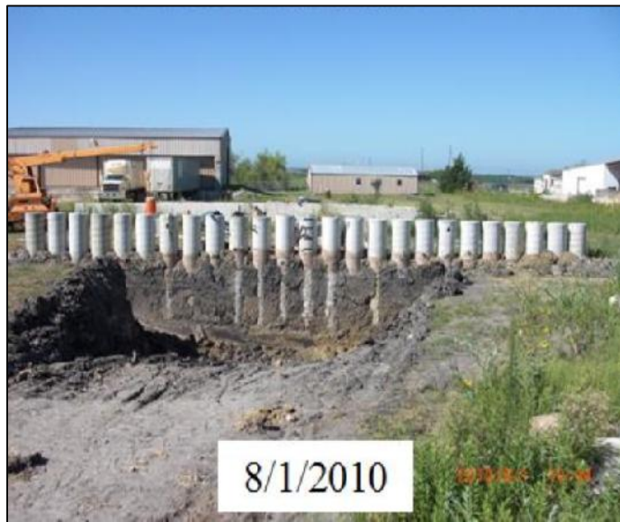
Figure 6.12: 1:1 Slope excavation to the depth of 9ft (8/1/2010)
