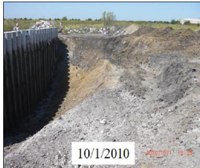
Figure 6.14: 3:2 Slope excavation to the depth of 15ft (10/1/2010)
