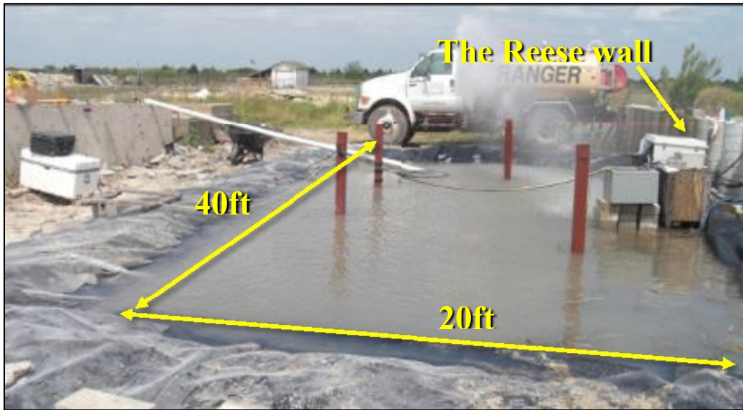
Figure 3.24: Inundation pond during wet conditions
