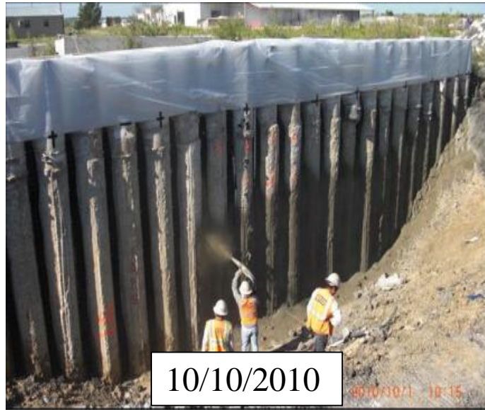
Figure 6.15: Shotcrete finishing of passive side (10/10/2010)
