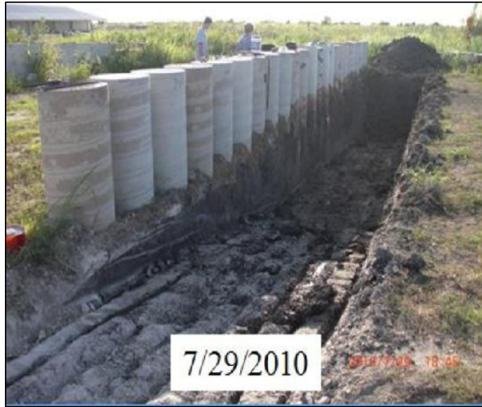
Figure 6.11: Excavation of 9ft deep trench (7/29/2010)
