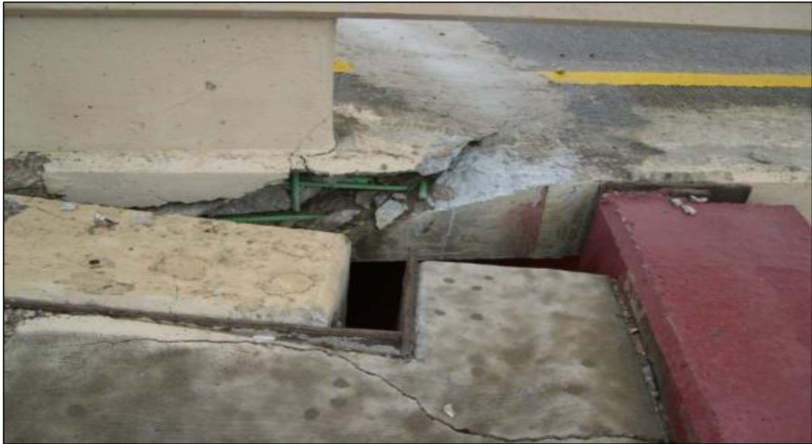
Figure 2.15: Wall failure during short-term conditions (Smith 2009)
