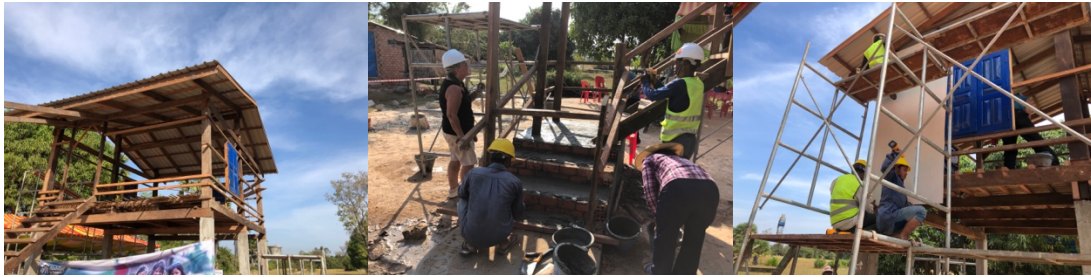
Figure 4: Day 4 Work Activities
