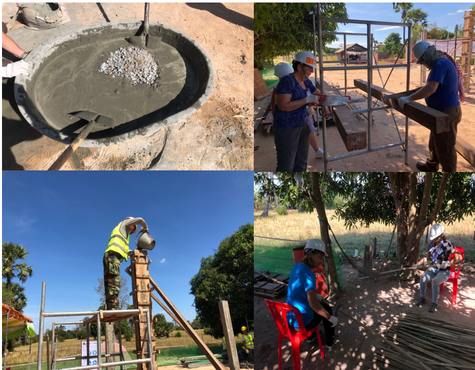
Figure 2: Day 1 Work Activities
