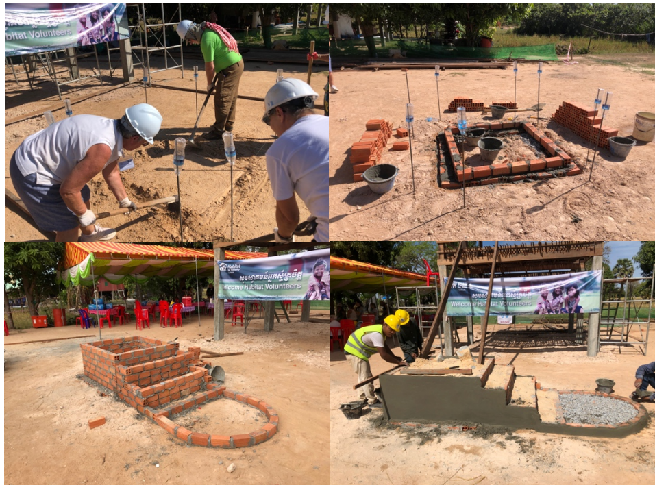
Figure 3: Construction of Stair Landing
