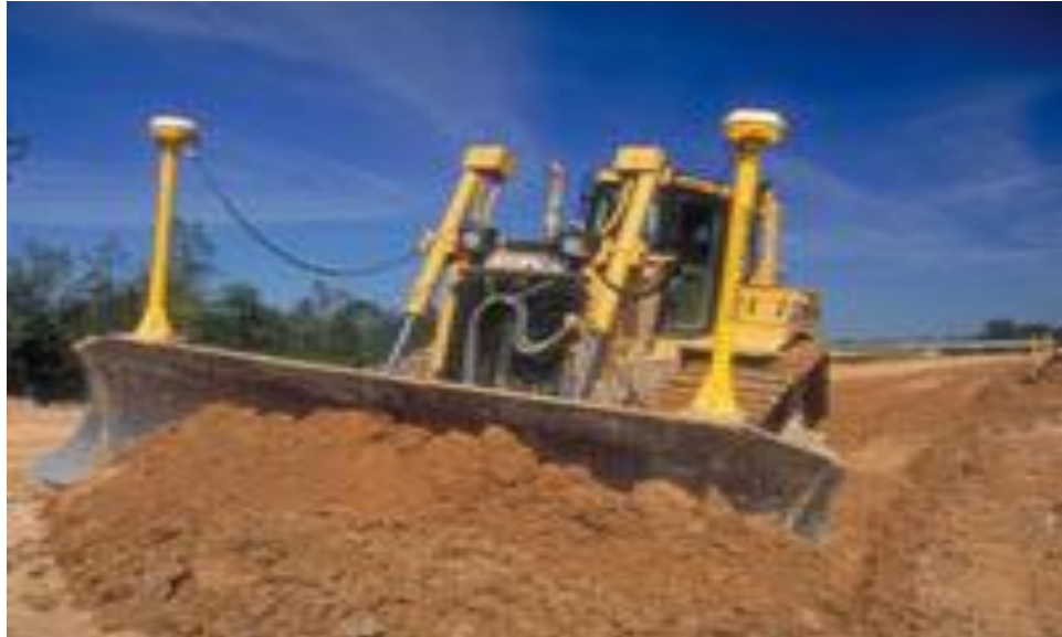
Figure E-1: Bulldozer excavating and spreading earthwork
