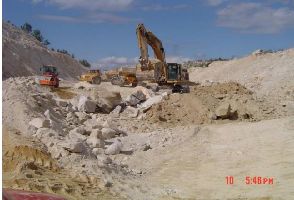
Figure E-3: Earthwork backfilling, loading and compacting operations
