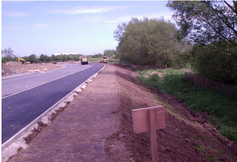
Figure E-5: Earthwork compaction on shoulder of bypass road in Middlesbrough
