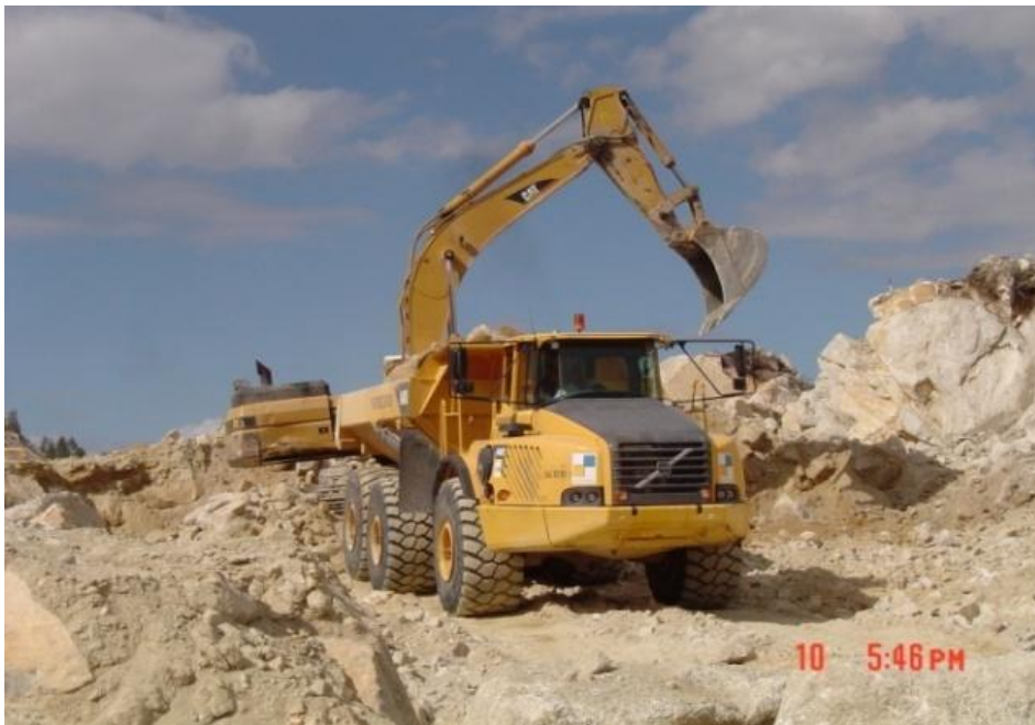
Figure E-4: Earthwork excavation and loading operation
