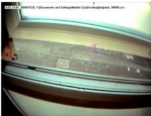
Figure 3.4 Participant (expert) examining window and observes force mark damage on the inside of the frame. Red-cross hairs suffering from drift however object is within the centre of the video frame.
