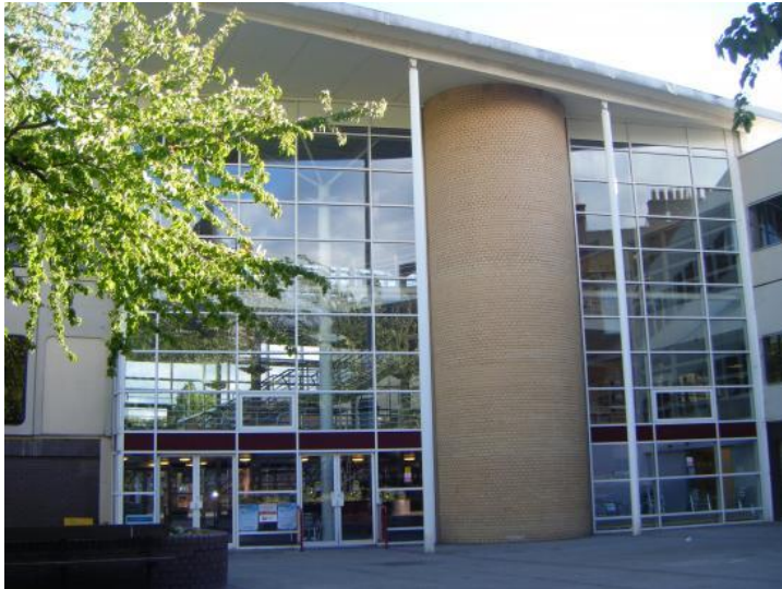
Figure 1: The Clarendon Building, Teesside University (Preston, 2019)
