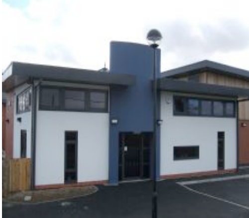
FIG. 8: Primary school main entrance
