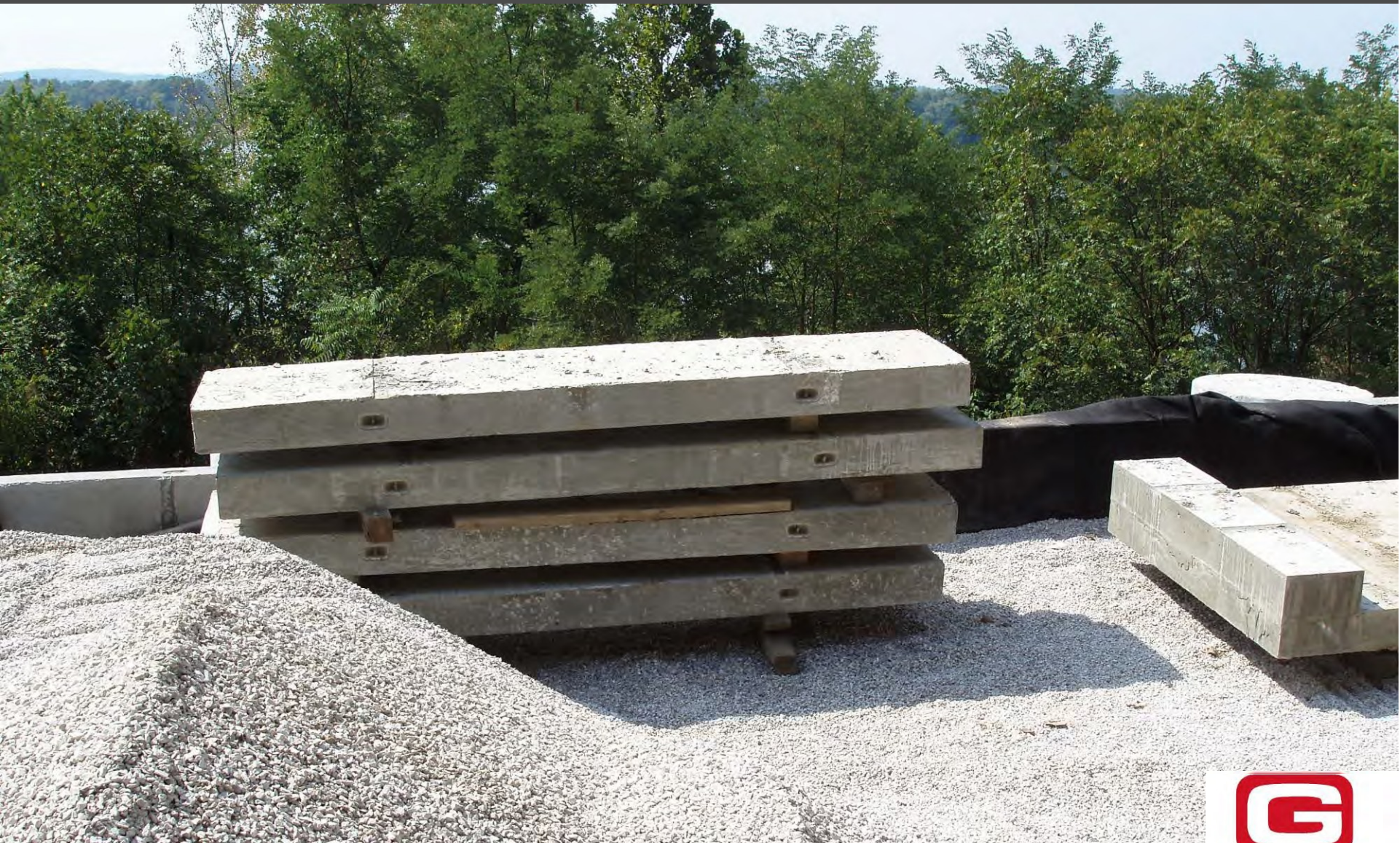
SR 66 Landslide, Perry County, Indiana
