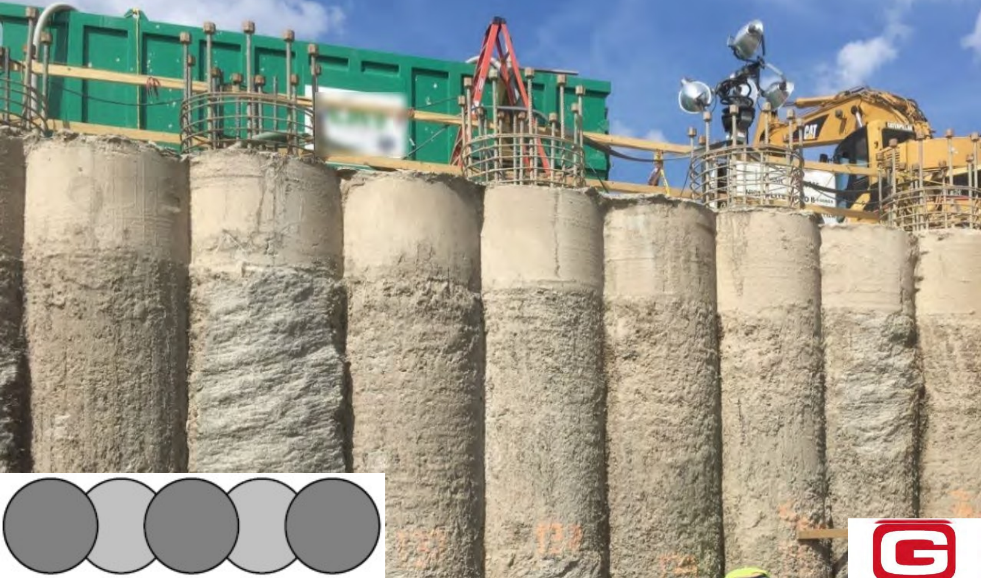
Drilled Shaft Secant Wall
