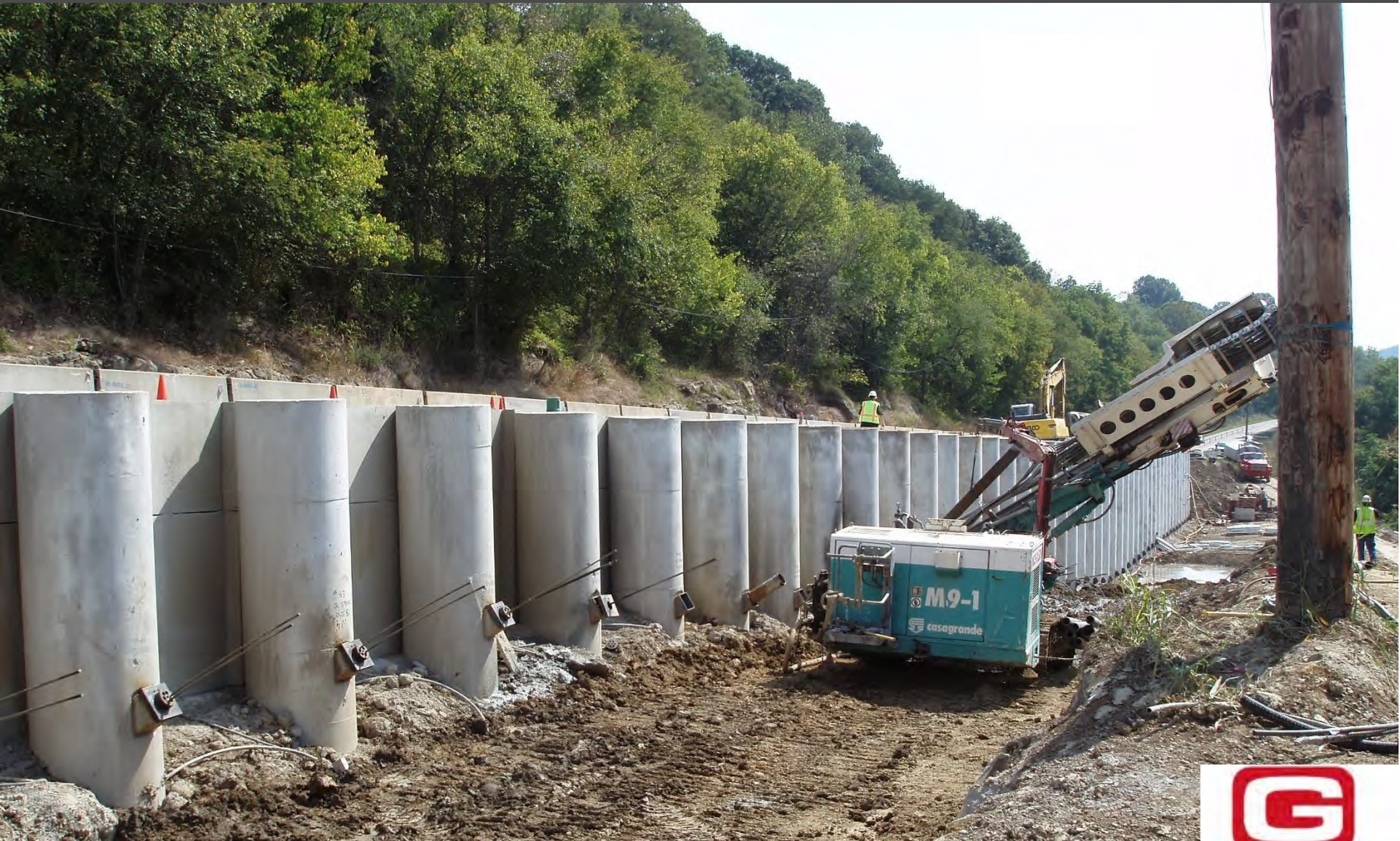
Drilled Shaft Wall with Tiebacks
