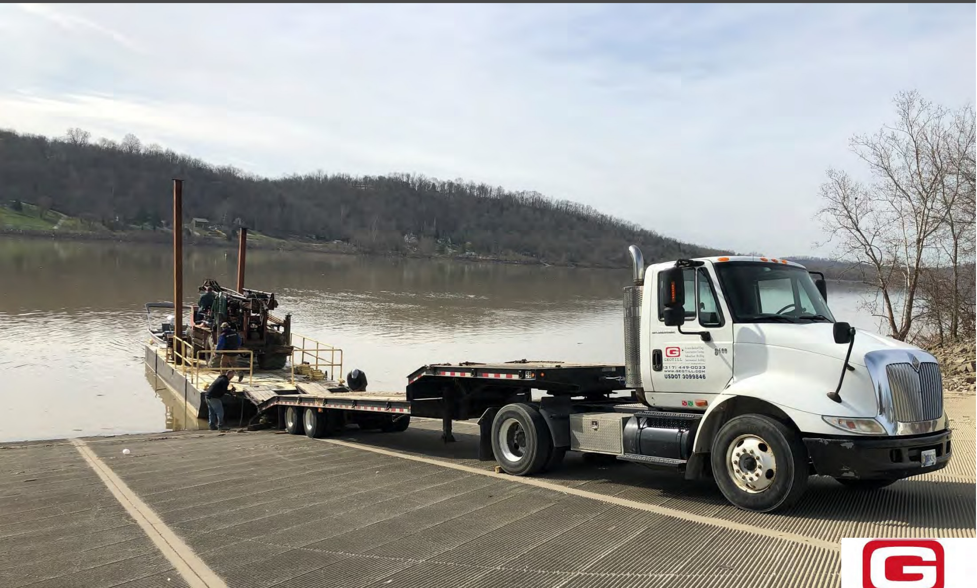
SR 156 Landslide RP 24.1 (Launching Rig in Ohio River)
