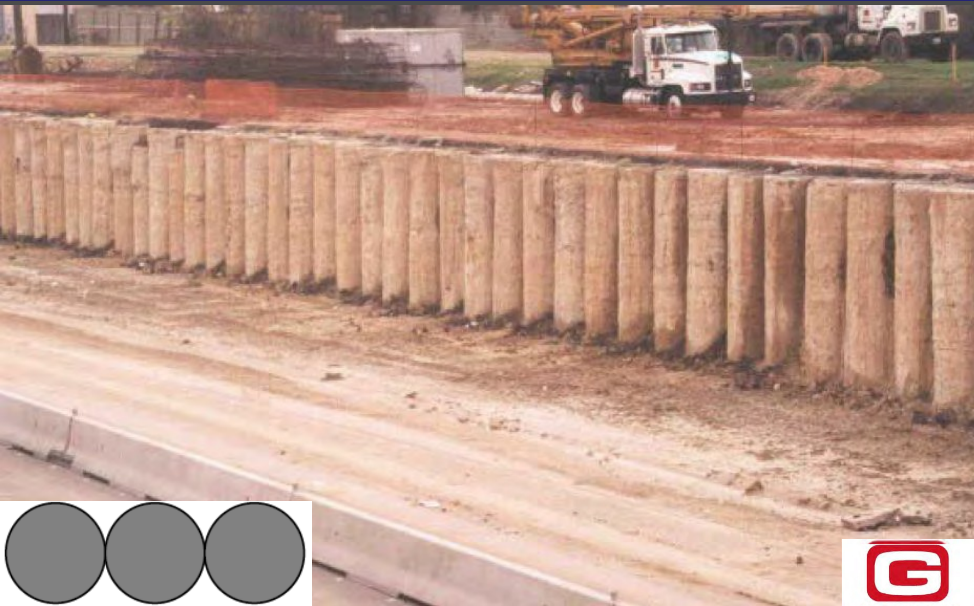
Drilled Shaft Tangent Wall
