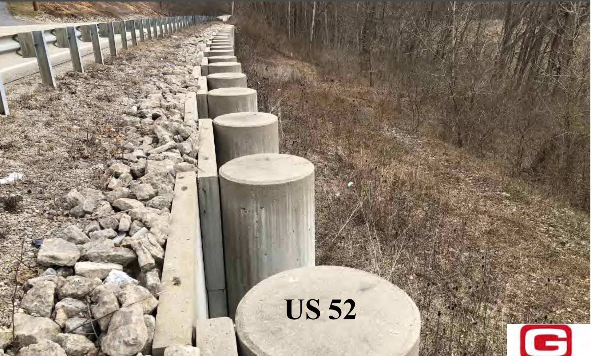
Drilled Shaft Wall with Lagging
