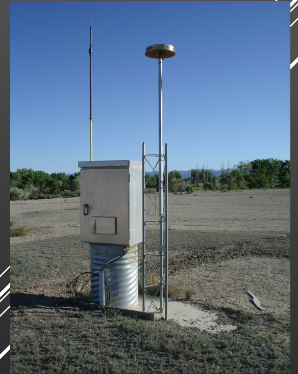
"CORS GNSS Reference Station." CORS GNSS Reference Station, 2013, emap.mesacounty.us/gps_survey/CORSMC03.htm .
