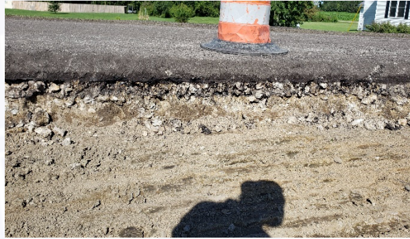
2019 - Patching location showing macadam layer with large aggregate
