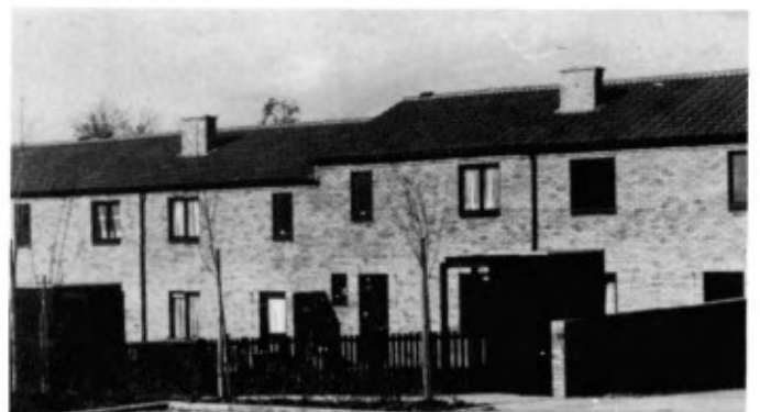
Downsbarn coal fired houses
