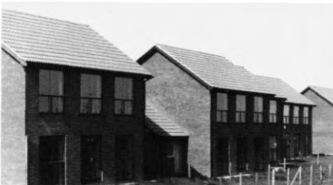
Great Linford low energy and passive solar houses
