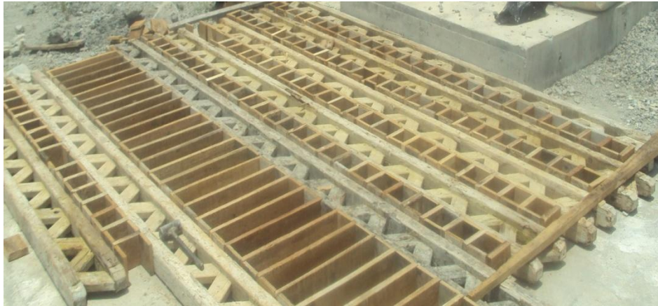
Figure. 3: Moulds for concrete cubes and beams
