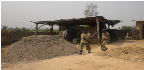
Figure 5: Blocks transported on pallets from production shed to curing section.
