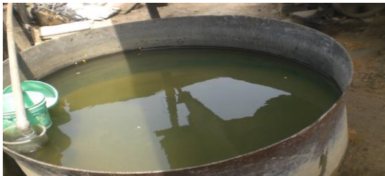
Figure 3: Water for works
