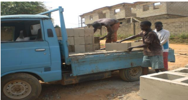
Figure 9: Offloading blocks for use on site.
