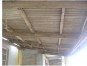
Plate 4.3.2: Roof Ceiling Showing Timber Trusses
