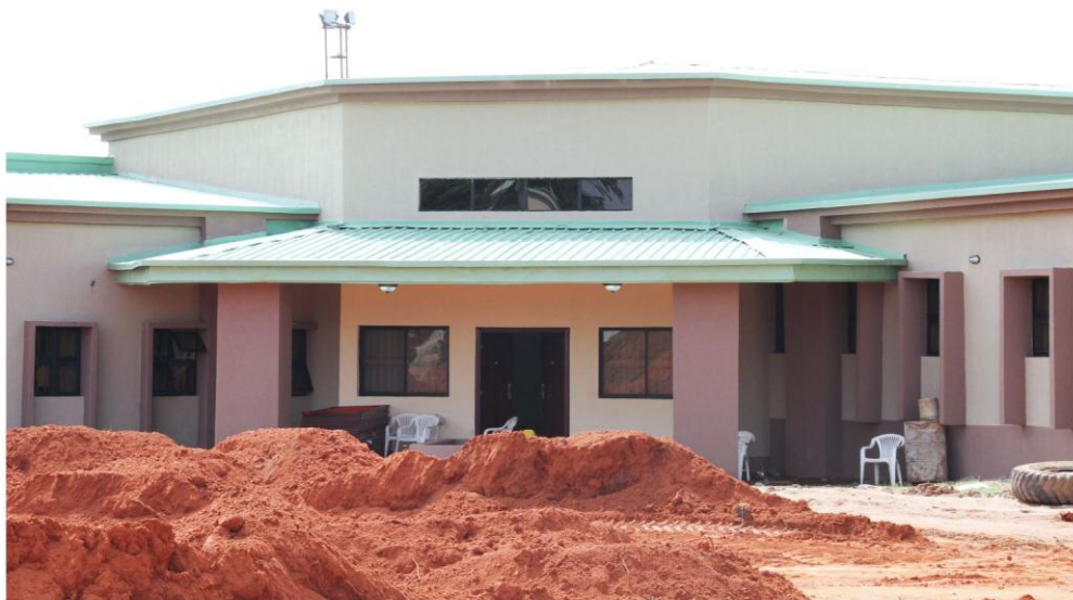
Construction site of Covenant University Secondary School
