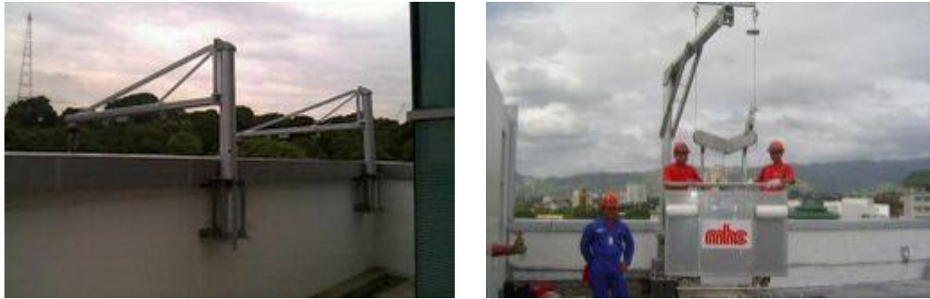
Figure 3a&b: Rigging system
