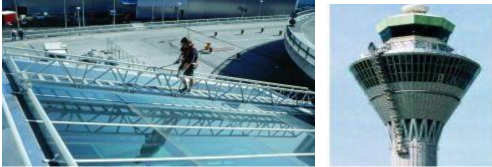
Figure 6a&b: Ladder and gantry system
