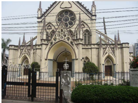
Plates 4.1.2: Entrance approach view of the reconstructed structure in 1932 (fieldwork picture 2007)
