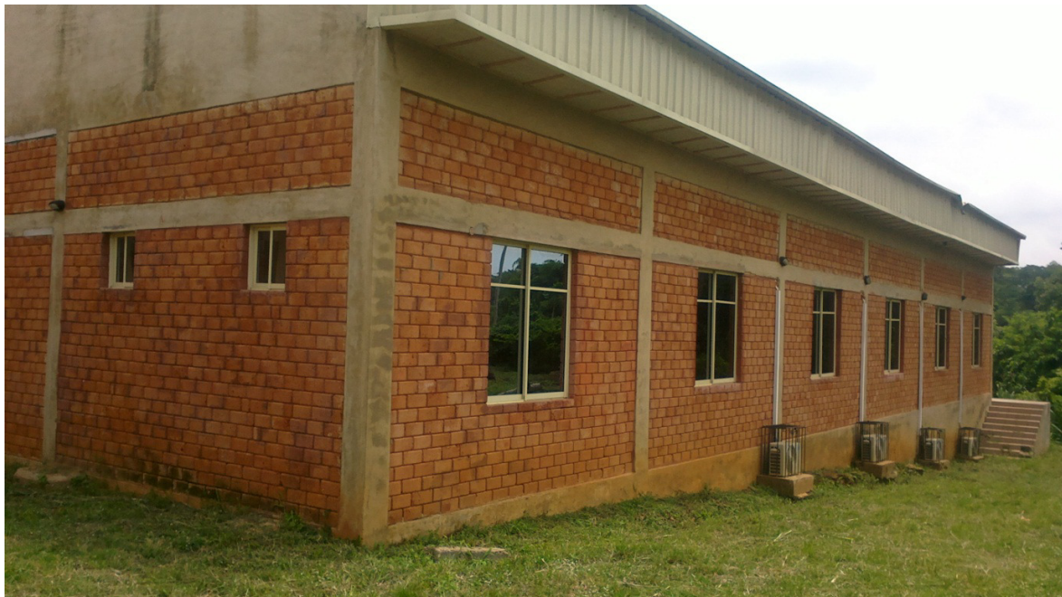
Figure 2: Electronics Testing Centre, Federal University of Technology, Akure, Nigeria was built in 2008 with stabilized interlocking blocks
