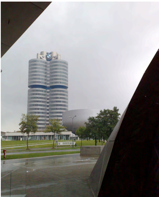
Photograph 17: Schwaner tower and the building as screen. (own picture)
