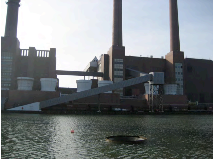
Photograph 23: The plant chimneys, seen from Autostadt (own photo)
