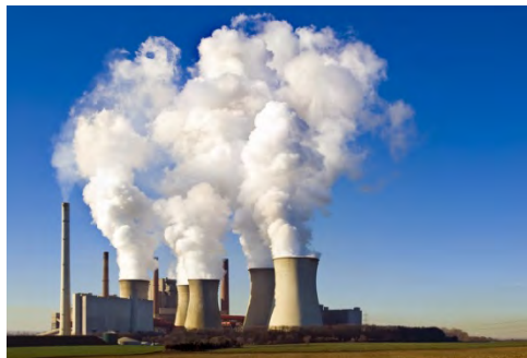
Flexible fossil fuel power plant
