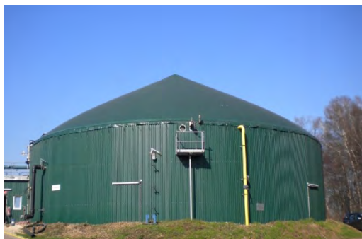
Load following Biogas power plants
