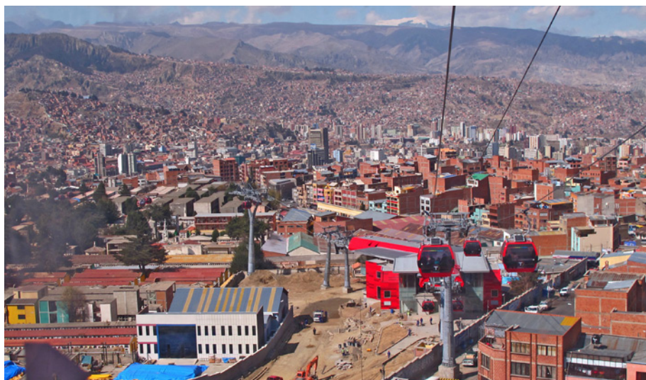
Figure 2: Construction without significant disruption of daily routine in La Paz, Bolivia
