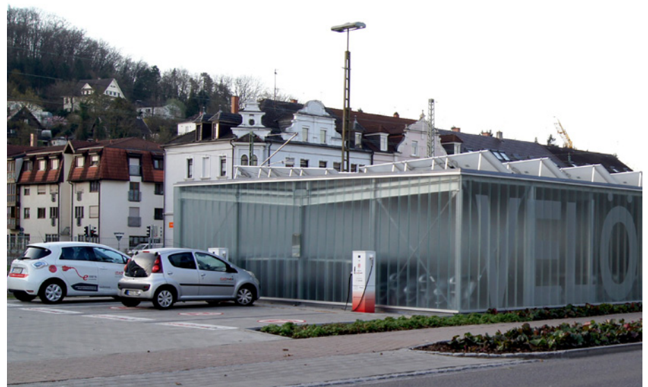
Figure 2: The Stadtmobil e-car sharing vehicles may be found at the new bicycle parking hall.
