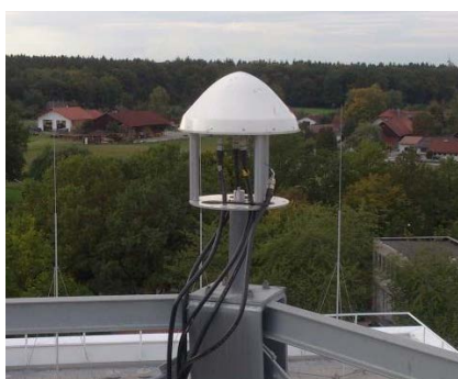
Figure 6: Roof installation of antenna array
