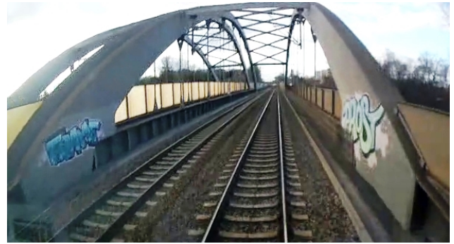
Fig. 7. Metallic railway bridge from train driver's perspective.
