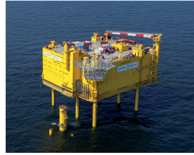
Figure 5: Helwin1 offshore platform.
